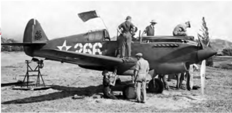
*This early P-40 is from the 18th Pursuit Group, and the ground crew is bore-sighting its twin nose-mounted .50-caliber machine guns at Bellows Field sometime in the summer or fall of 1941. This procedure ensures the guns' bullets converge at a desired range.*
