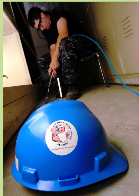
US Navy Photo by MCSN Donald White Machinist Mate Fireman James Knowlton uses a needle gun to remove the tile from the deck June 8 in preparation for new flooring to be installed.
