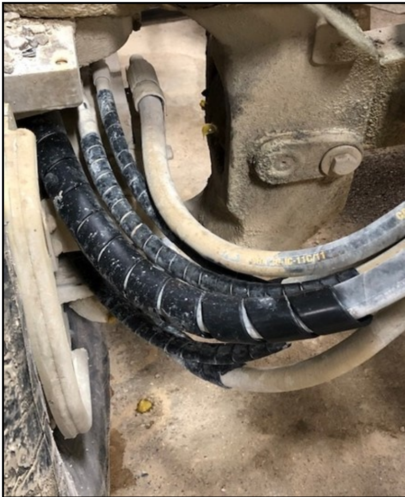
Spiral wrap on road grader's front hydraulic drive.
