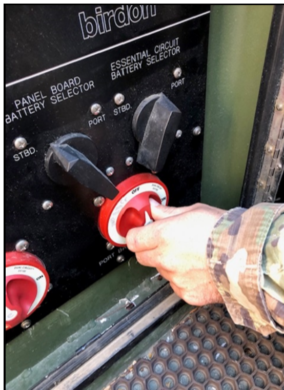
Turn OFF batteries on the starboard (right) side of the BEB.
