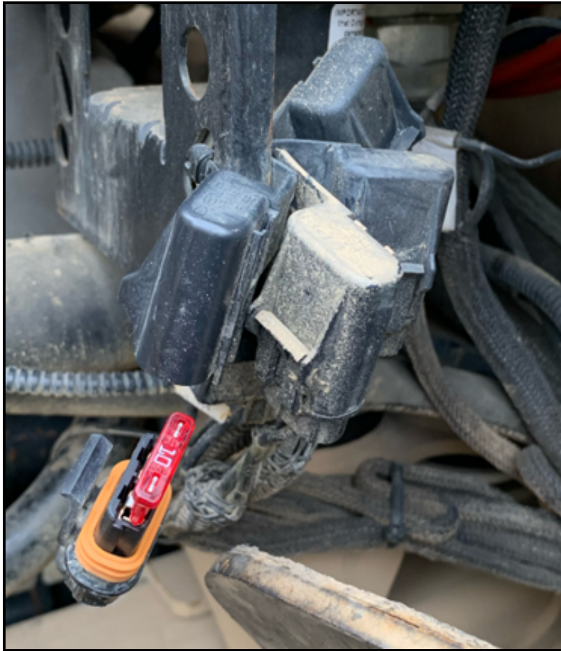
10-AMP fuse on C51 connector with fuse cover removed
