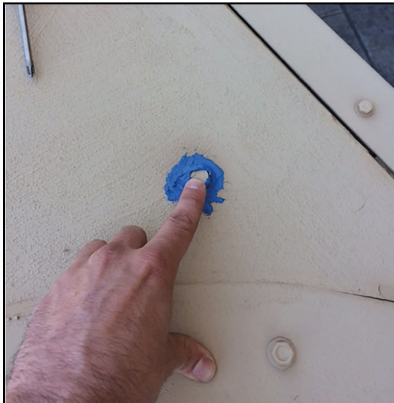
Adhesive silicone seals out water
