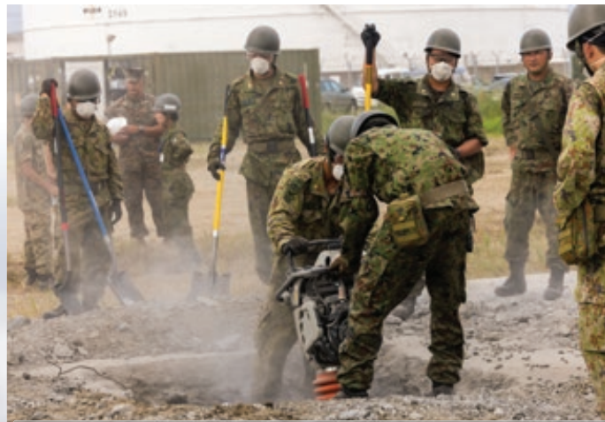
クレータ技術を練習する、第13施設隊の陸上自衛隊員。 Service members with the 13th Engineer Brigade, Japan Ground Self-Defense Force, practice cratering techniques.
