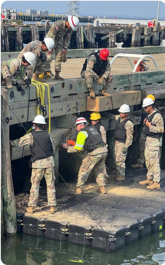
**Soldiers deconstruct damaged sections of a pier.**
