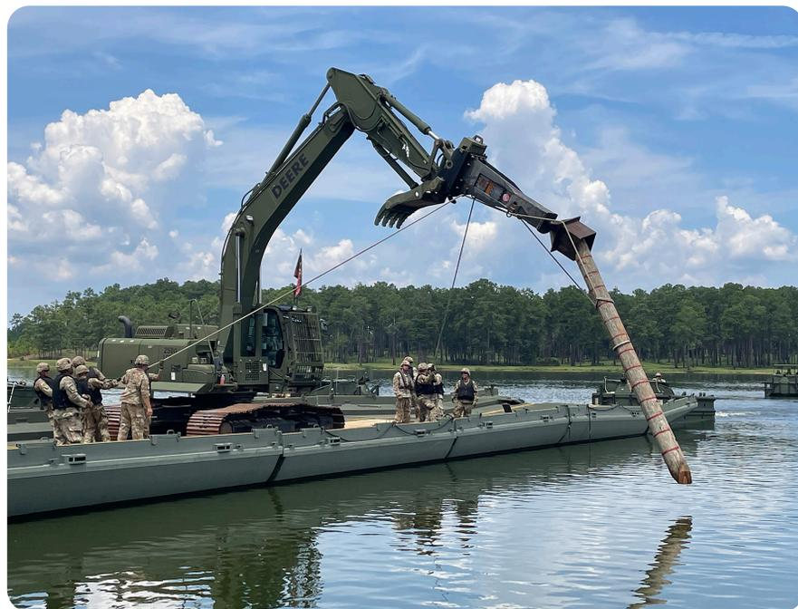
**The 554th ECC and the 497th MRBC move a timber pile into place to test pile driving from an IRB.**
