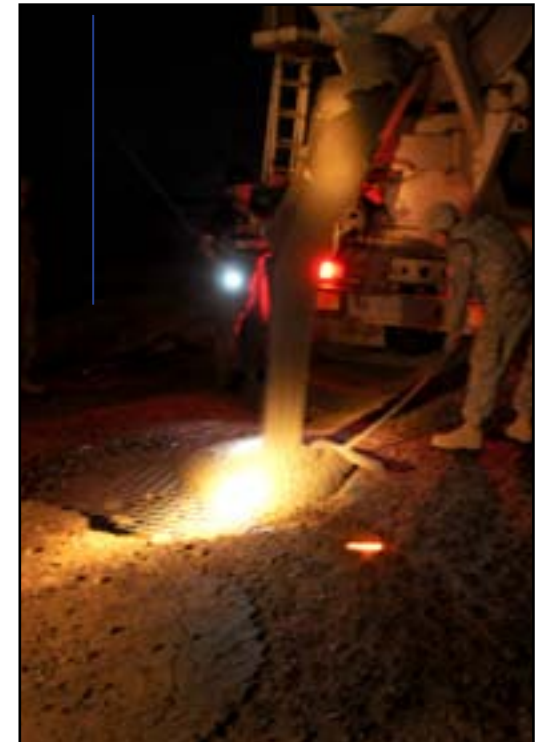
A Soldier with 3rd Platoon, 573rd Clearance Company, 1st Engineer Battalion, spreads out cement and maintains proper filling measurements during a crater repair mission, June 25, in Salah-ad Din province, Iraq.
