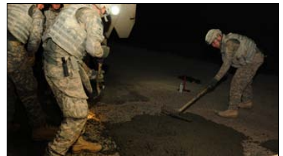
Private First Class Spencer Haines, a combat engineer, with 3rd Platoon, evens out recent cement filling with the help of other Soldiers in his unit during a crater repair mission, June 25.
