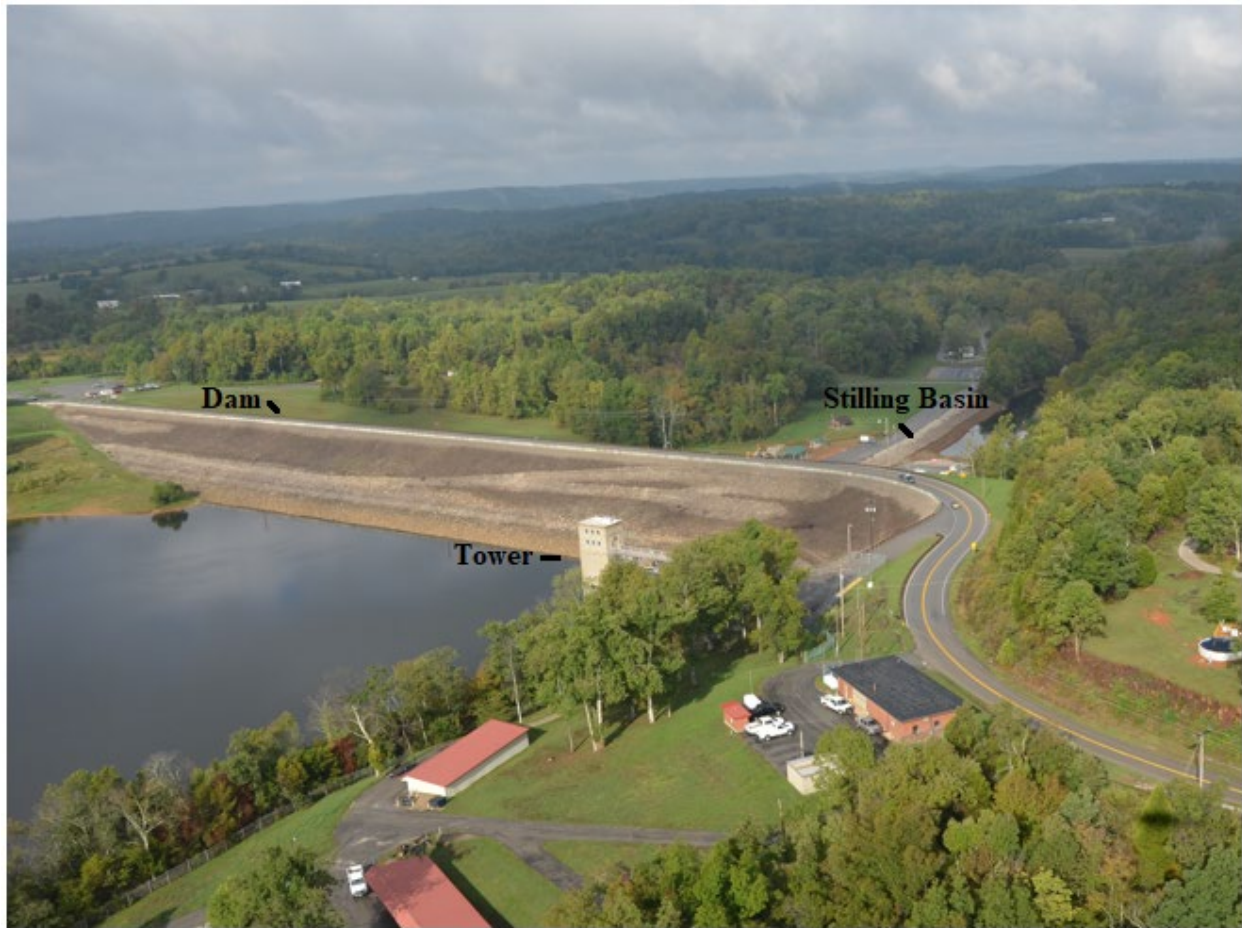
Figure 2- Operating tower and outlet works at Rough River Lake Dam.
