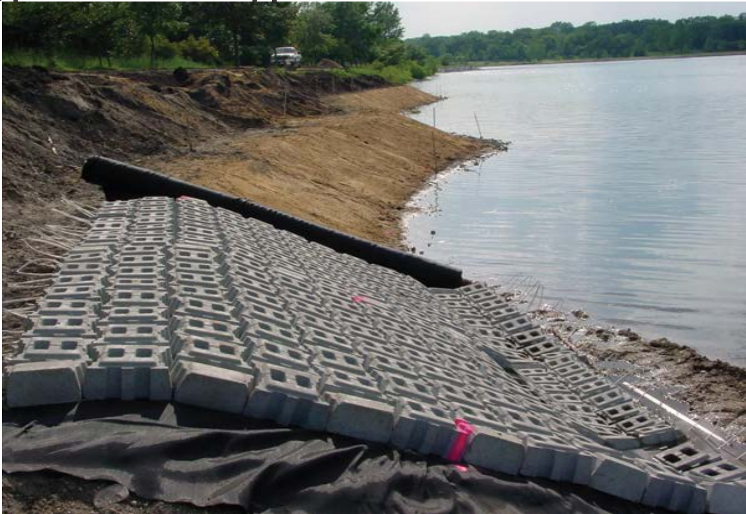
Photo Showing Installation of Articulated Concrete Revetment
