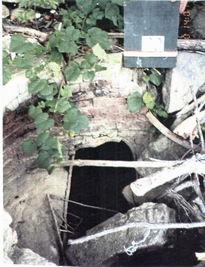
18" OUTFALL INSIDE COLLAPSED MANHOLE
