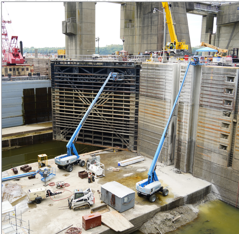
The Great Lakes and Ohio River Division's Regional Rivers Repair Fleet work to rehab the miter gates in the 1,200-foot lock chamber at John T. Myers Locks and Dam on the Ohio River, Sept. 12, 2023.
