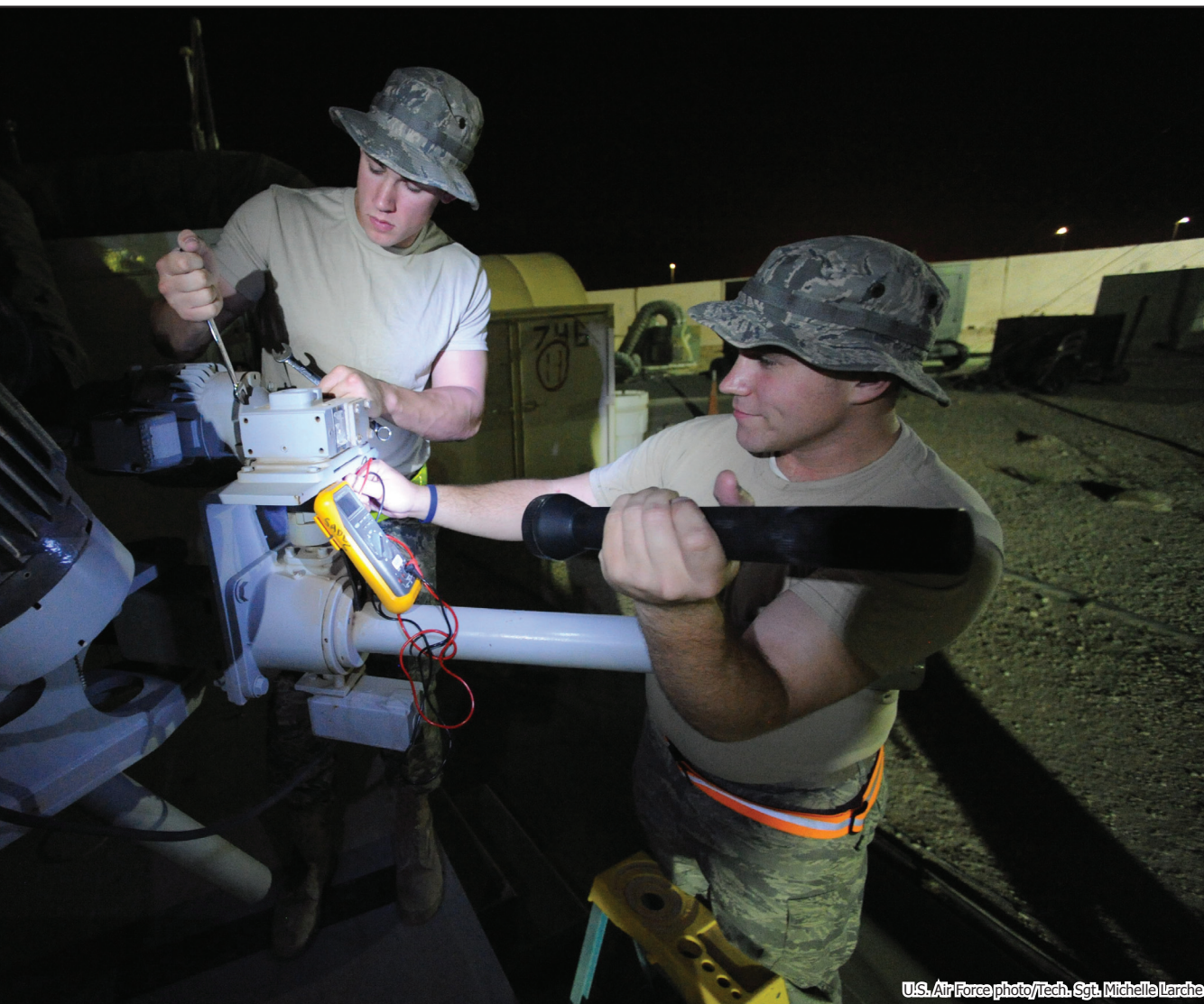
TOP RIGHT: Senior Airman Sean Brewer (left) and Staff Sgt. Sean Collins, 379th Expeditionary Operation Support Squadron link maintenance, adjust an antenna's azimuth and elevation motors here, June 14.
