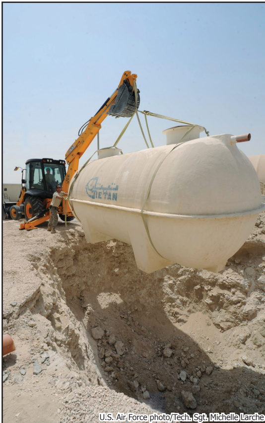
BOTTOM LEFT: Staff Sgts. William Walker and Donald Berendt, 379th Expeditionary Civil Engineer Squadron heavy equipment, use a backhoe to lower a new cadillac waste tank here, Wednesday.
