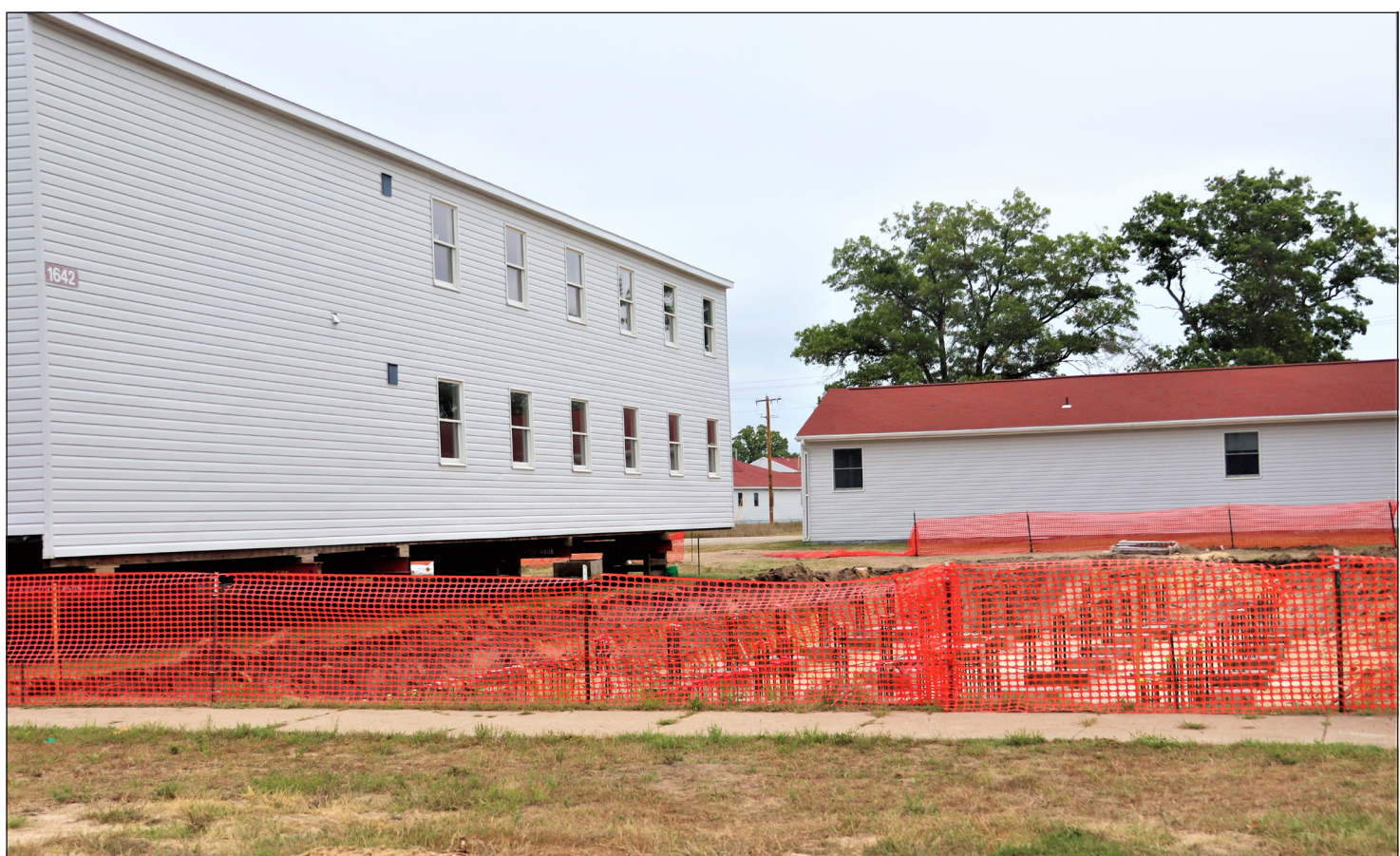
(Above and below) The construction area for a new foundation for a World War II-era barracks is shown Sept. 6 at Fort McCoy. The work is the next step after four World War II-era barracks were relocated from one block on the installation to new locations on post and have to be reset at their new locations with new foundations, utilities, etc. The effort to relocate barracks buildings in 2023 was the first time that effort was ever completed in Fort McCoy's history.
