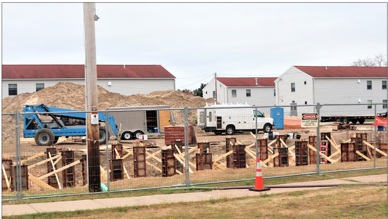
(Above and below) The construction area for a new foundation for a World War II-era barracks is shown Sept. 6 at Fort McCoy. The work is the next step after four World War II-era barracks were relocated from one block on the installation to new locations on post and have to be reset at their new locations with new foundations, utilities, etc. The effort to relocate barracks buildings in 2023 was the first time that effort was ever completed in Fort McCoy's history.
