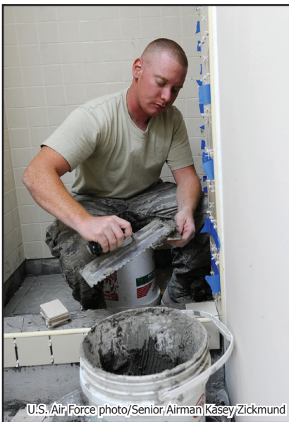
BOTTOM LEFT: Airman 1st Class Kevin Strickland, 379th Expeditionary Civil Engineer Squadron heating, ventilation, and air conditioning journeyman, adds adhesive to a ceramic shower tile here, Thursday.
