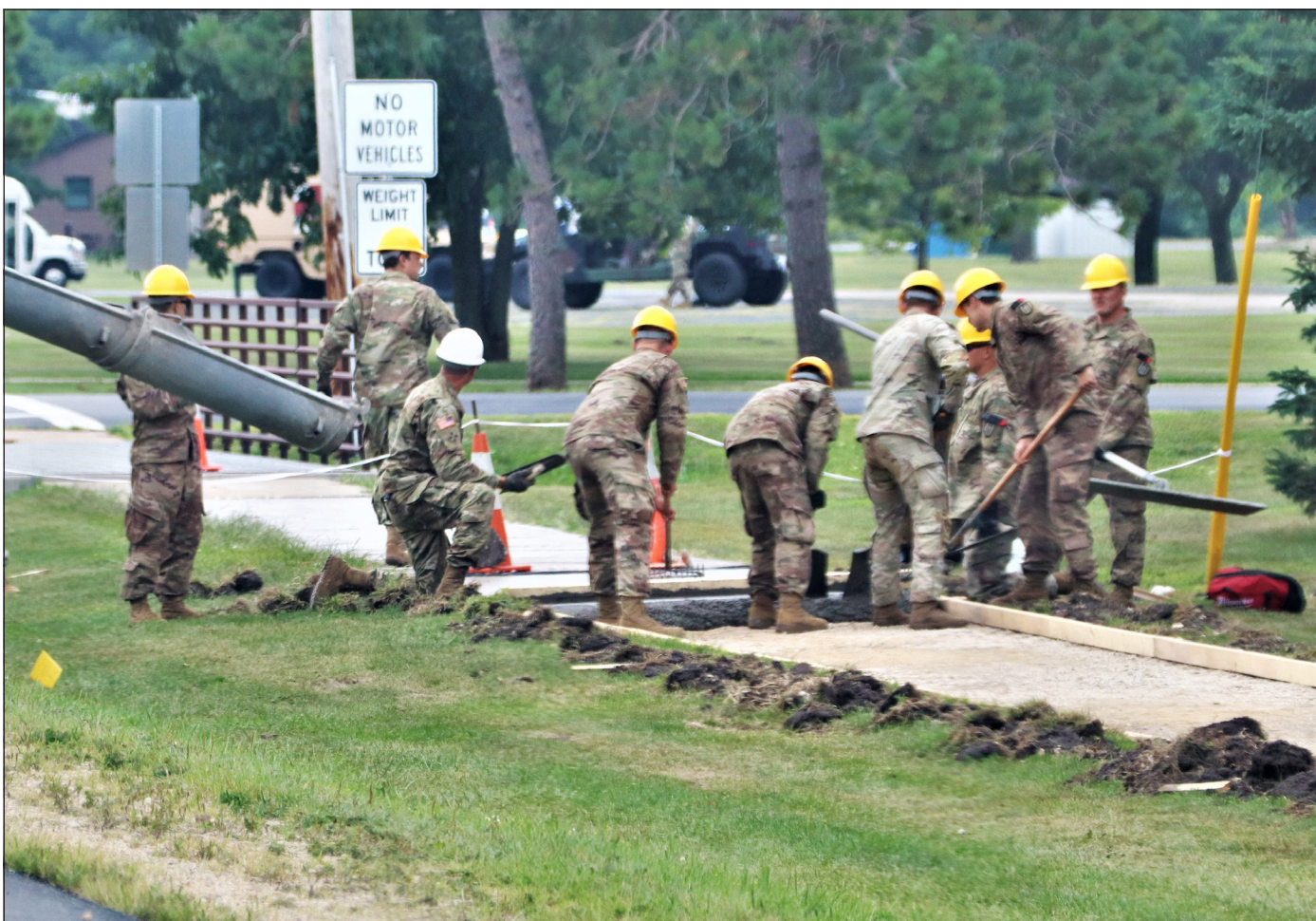
Soldiers with the 996th Engineer Company, an Army Reserve unit based in Milwaukee, work on a troop project to replace a section of sidewalk Aug. 21 on the cantonment area at Fort McCoy.
