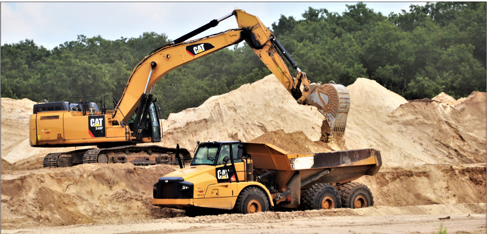
(Above and below) Contractors move dirt from a borrow pit Aug. 2 next to the cantonment area fence at Fort McCoy, Wis. The location has also been a spot for an ongoing troop project on post for the past two years. The dirt movement was to an ongoing construction project on the installation.
