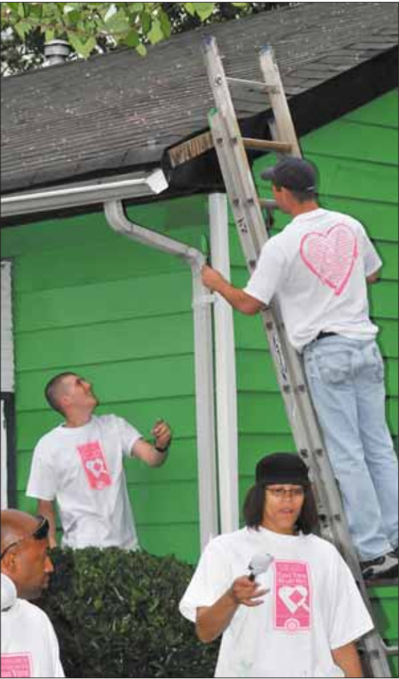
Sailors from Naval Medical Center Portsmouth paint the home of Portsmouth resident Carrie Gaines as part of the April 17 community relations project, “Paint Your Heart Out.” The event, sponsored by the Portsmouth Rotary Club, helps low-income, disabled and elderly homeowners with upkeep they can no longer handle on their own. Some 119 NMCP service members painted, weeded, landscaped and removed debris from two homes selected for the event.
