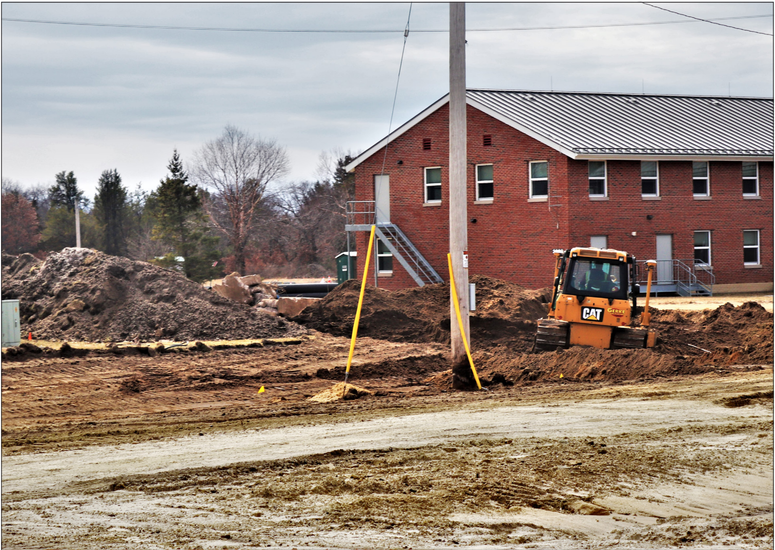
Work as part of an $850,000 grading project is shown April 3 (above) and April 19 (below) on the cantonment area at Fort McCoy. An extensive grading project began in April 2023 around Fort McCoy's building 2000 on the cantonment area to improve drainage in that area, according to the Fort McCoy Directorate of Public Works. The project was awarded to RHI Construction, and Gerke Excavating of Tomah, Wis., is working as a subcontractor on the project. The work comes just several years after building 2000 itself was upgraded in 2018-19 with an approximate $5.1 million renovation. The project's completion is expected to be summer 2023.
