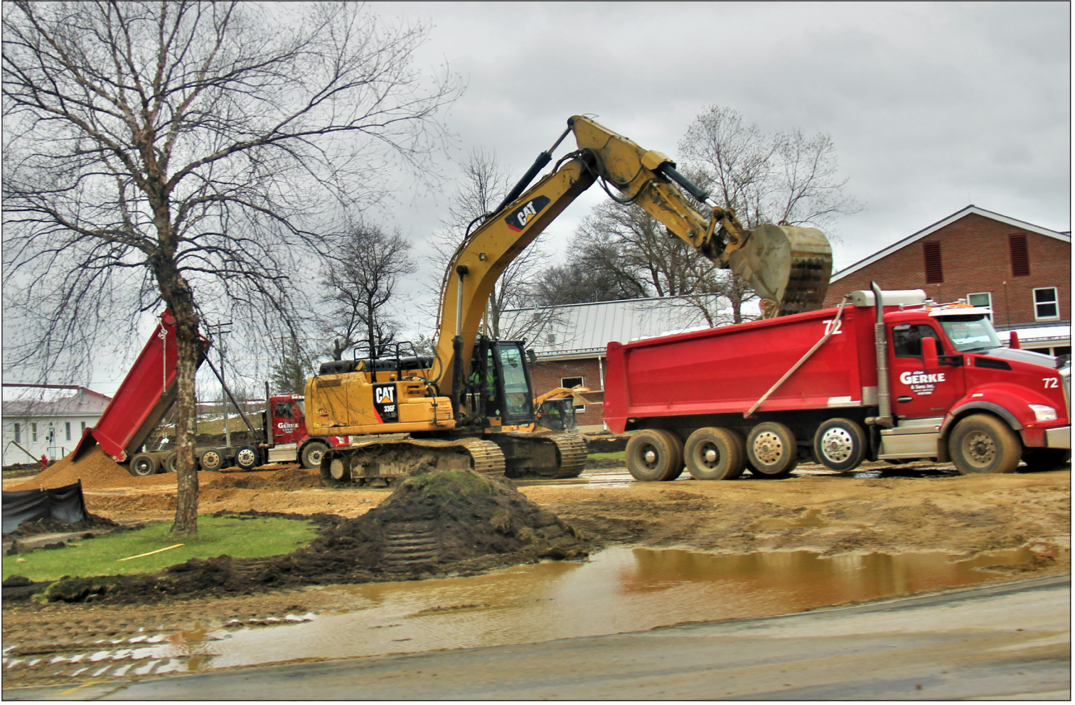
Work as part of an $850,000 grading project is shown April 3 (above) and April 19 (below) on the cantonment area at Fort McCoy. An extensive grading project began in April 2023 around Fort McCoy's building 2000 on the cantonment area to improve drainage in that area, according to the Fort McCoy Directorate of Public Works. The project was awarded to RHI Construction, and Gerke Excavating of Tomah, Wis., is working as a subcontractor on the project. The work comes just several years after building 2000 itself was upgraded in 2018-19 with an approximate $5.1 million renovation. The project's completion is expected to be summer 2023.
