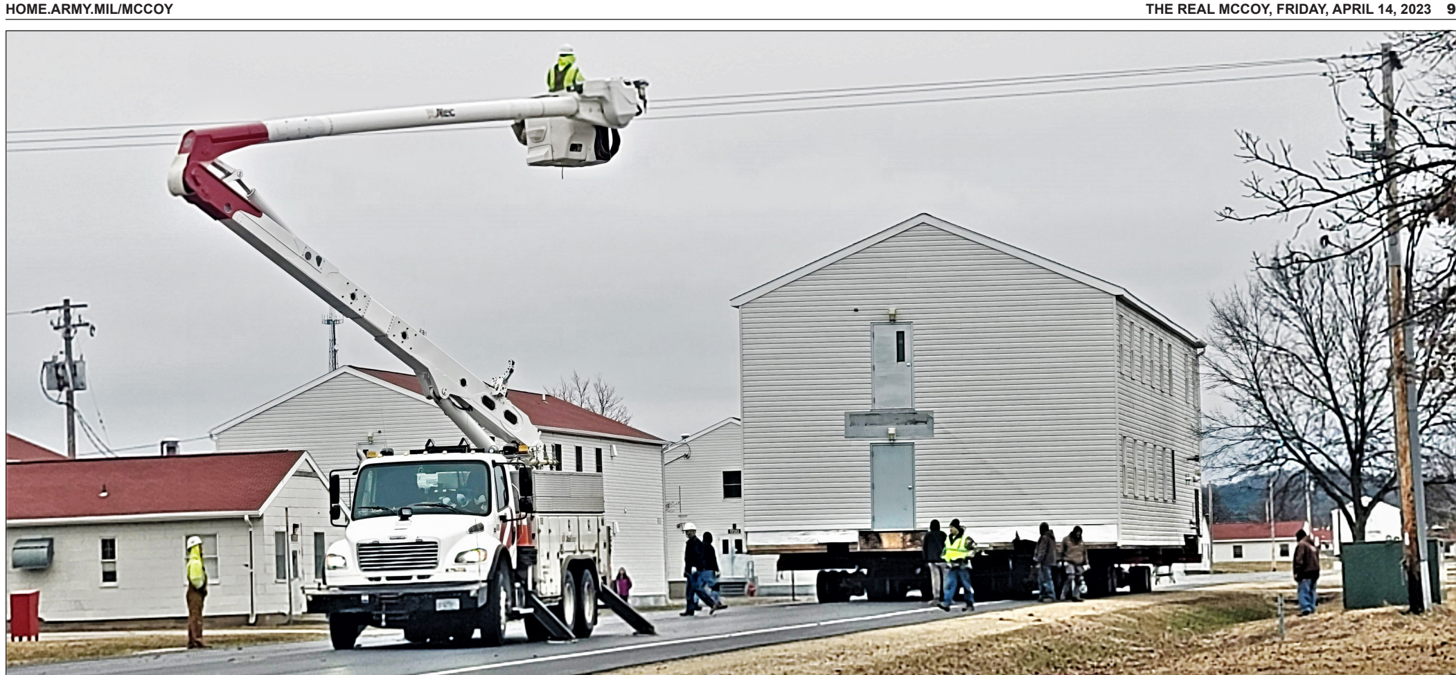
Contractors with JMJ Construction of New Lisbon, Wis., along with support from Heritage Movers of Blue River, Wis., move a third World War II-era building from the 1600 block on the cantonment area to the 1800 block April 4 at Fort McCoy.
