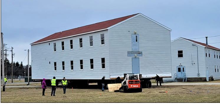
(Above, below left, and below right) Contractors with JMJ Construction of New Lisbon, Wis., along with support from Heritage Movers of Blue River, Wis., move the third World War II-era building into its spot in the 1800 block April 4 at Fort McCoy.
