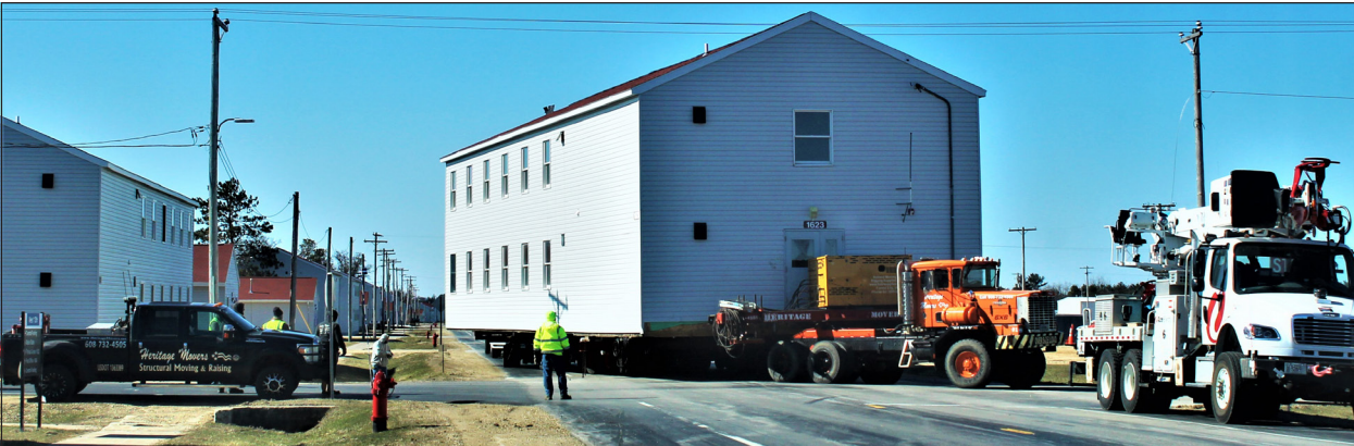
Contractors with JMJ Construction of New Lisbon, Wis., along with support from Heritage Movers of Blue River, Wis., move the fourth World War II-era building from the 1600 block to the 2800 block April 6 at Fort McCoy.
