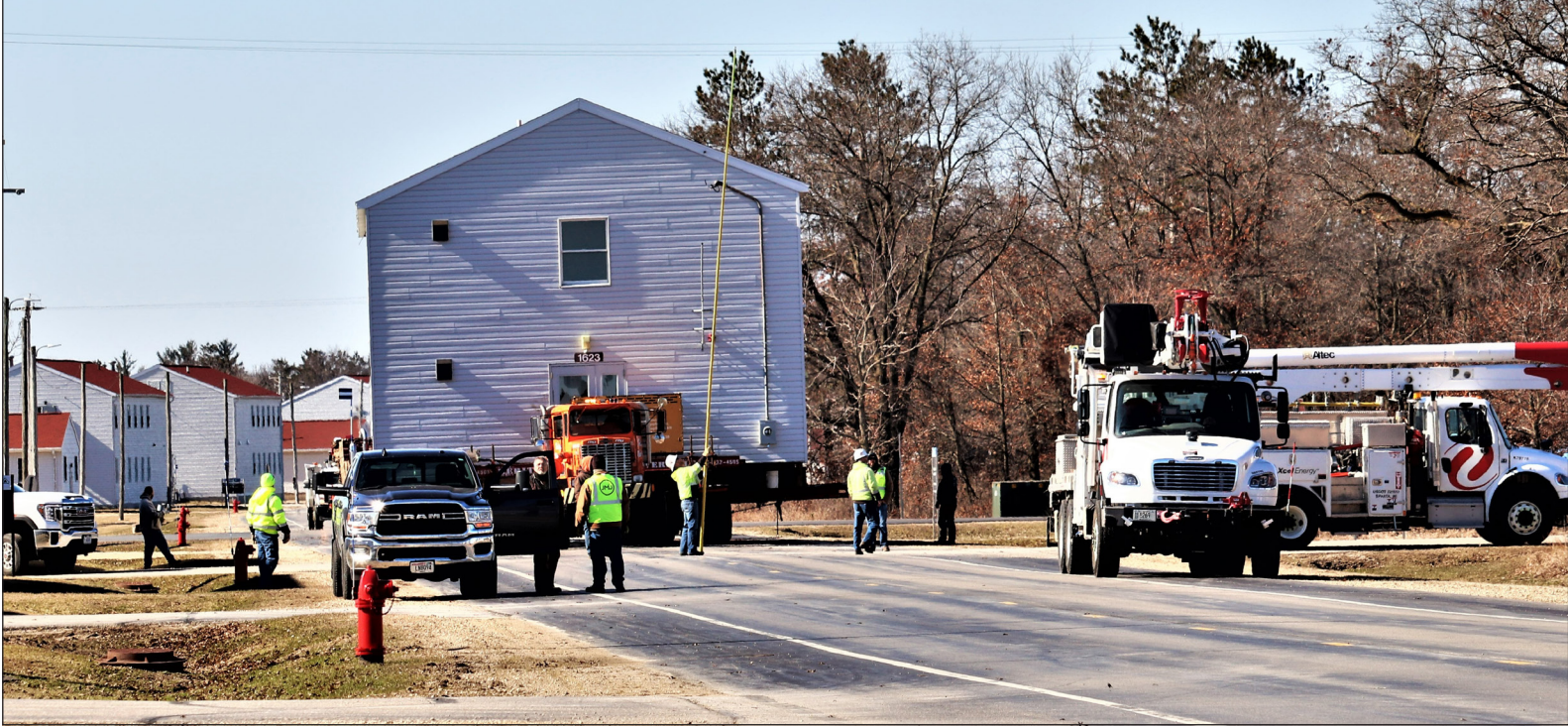
(Above and below) Contractors with JMJ Construction and Heritage Movers move the fourth World War II-era building down the street from the 1600 block 2800 block April 6 at Fort McCoy. They had to carefully make their way under many sets of electrical wires along the way.
