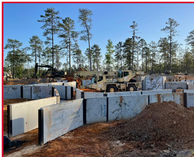
A crane emplaces the final walls.
