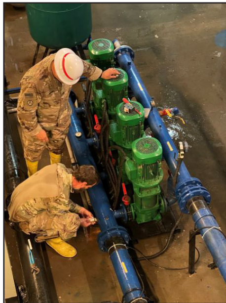
A Soldier assists an environmental engineer from the U.S. Army Corps of Engineers while he works to get the pumps back online at the water treatment plant.
