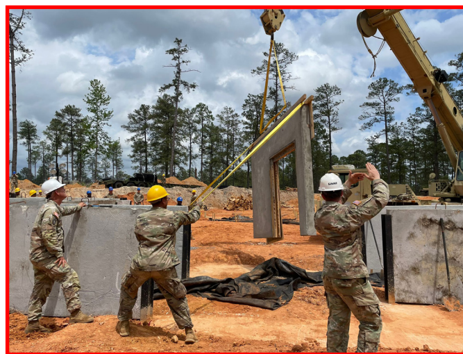
A Soldier serves as a ground guide for the crane operator while other Soldiers assist in emplacing bunker walls.
