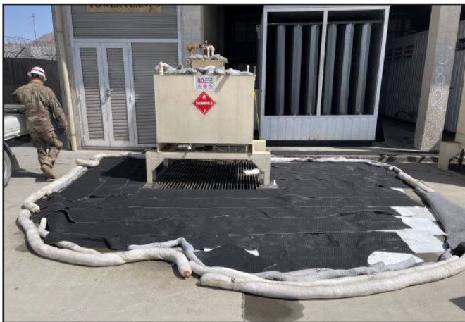
Containment material was placed on the ground to soak up the excess fuel after the generator day tank overflowed.
