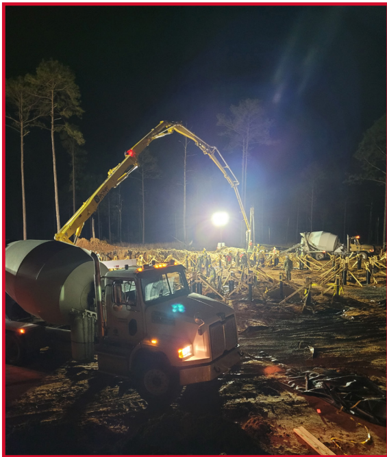
Concrete being poured for the I-beams and bunker footers
