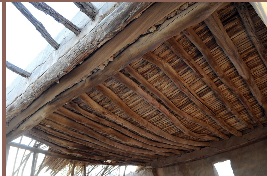
The roof of an old home (circa 1960s) in Al Rayyan, Qatar, March 19. The ceiling consisted of round timbers, roughly three inches in diameter. Mangrove slats ran perpendicular to the rods. A mangrur, matting woven with palm fronds, was rolled over the framework. Finally, a mixture of straw and mud, using well water, was poured on top. (Official Army Photo/Dustin Senger)
