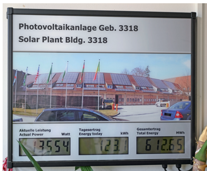
A panel in the DPW building counts how much electricity the panels on the roof of building 3318 are generating.
