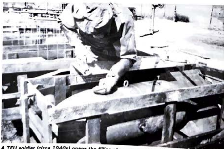
A TEU soldier (circa 1940s) opens the filling plug on a German mustard bomb to drain the agent into one-ton containers.
