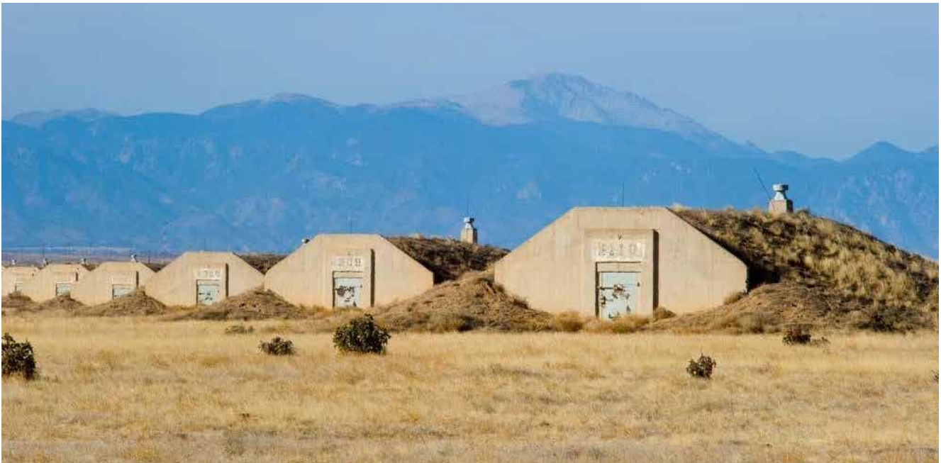
CMA is responsible for the safe and secure storage operations at the Army’s two remaining chemical weapons stockpile sites located at Pueblo Chemical Depot, Colorado, and Blue Grass Chemical Activity at Blue Grass Army Depot, Kentucky. (U.S. Army photo)
