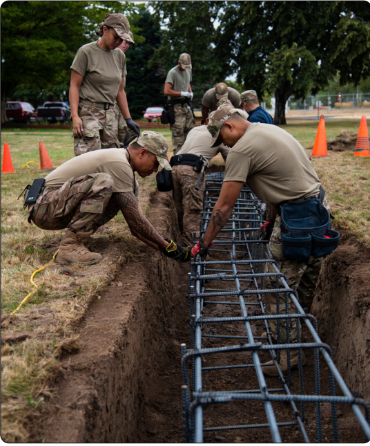
Photo by Master Sgt. Steph Sawyer 142nd Wing Public Affairs Members of the Hawaii Air National Guard lay rebar in preparation for pouring concrete during annual training at Portland Air National Guard Base, Ore., on August 10, 2022.
