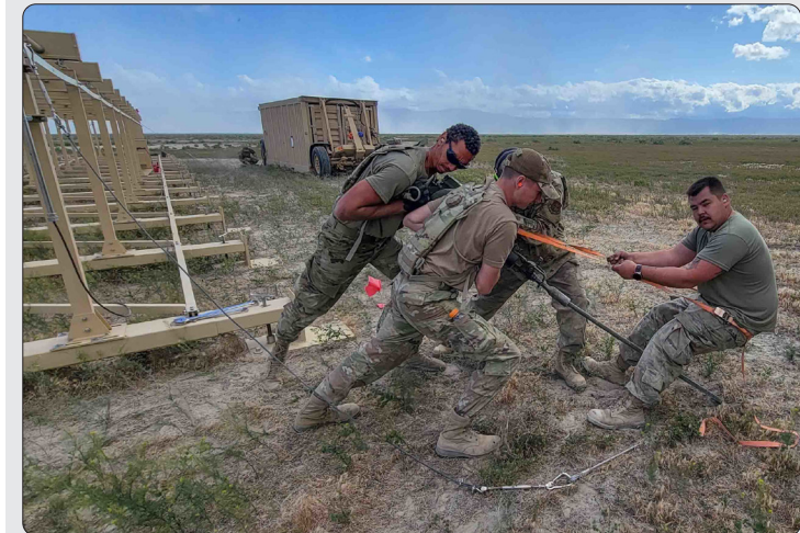
Courtesy photo by Master Sgt. Timothy Lombardi U.S. Air Force Staff Sgt. Loren Meeker (right) helps Airman 1st Class Jason Sharrer and Max Empol, and Tech. Sgt. Jay Hester drive a grounding rod into the soil as they set up equipment to create an active airfield during annual training at Amedee Army Airfield.
