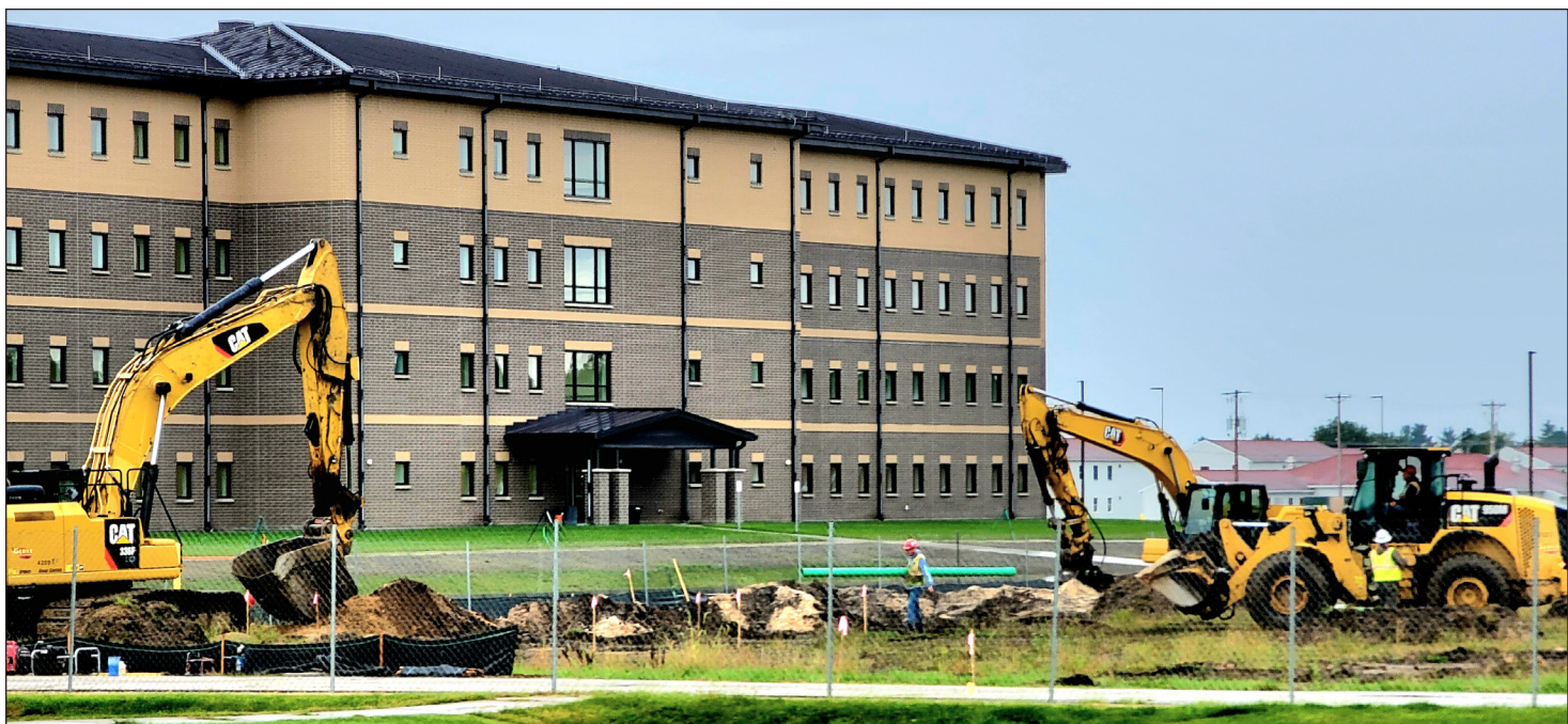
The construction area for a future transient training brigade headquarters in the 1600 block on the cantonment area is shown Sept. 12 (above) and Sept. 9 (below) at Fort McCoy. This early work was for the installation of a sewer system for the new facility.
