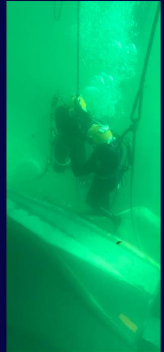
A 77,000-pound lift bag was suspended directly above the vessel, with two 10-ton chain falls attached to the lift bag's bottom by a strong back. ND2 Cayman Conley and ND2 Owen Craffey installed two 6,500-pound lift bags, one forward and one aft, to reduce overall weight and increase mechanical advantage for the Salvors to right the tug vertically for a much safer and more controlled lift.
