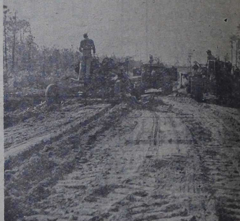
LEVELLING—Two 18-ton bulldozers and a towed road scraper level the earth dumped by the trucks. At the present time the approximately one-third completed (Official USMC Photo).
