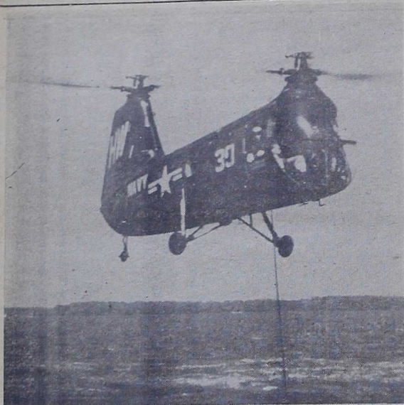
HUNTER-KILLER 'COPTER —A Navy HUP Piasecki helicopter hovers over the ocean surface while a sonar ball suspended from the cable in center probes the sea for submarines. Under study as a submarine hunter weapon for the past two years, the helicopter, which also has been tested with sub attack gear, is designed to screen the waters in advance of a convoy or other ship movement, hovering motionless through the use of an automatic pilot. Note a pilot leaning from the window as the craft flies "no hands."
