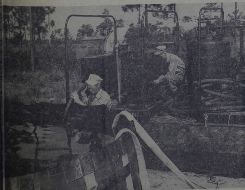
ENGINEERS BOTHER THIS STILL because use is to provide up to 1,500 gallons of water a day for troops in the field. Pfc Jim Varnadore, left, and Pfc Jerry Padden test the unit in a pre-field water drill . . .
