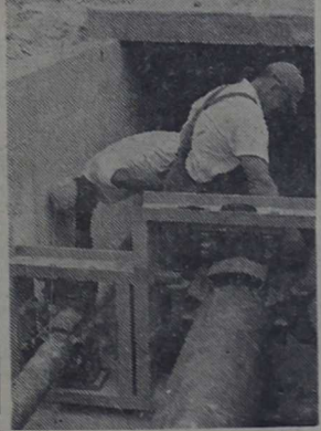
TUNNELWAY—Pipefitter Charley Haynes, of Birmingham, Ala., and Elwood Henderson, of Wallace, N. C., swab protective asphalt paint on steam pipes in the new pipe-system under construction here (Official USMC Photo).
