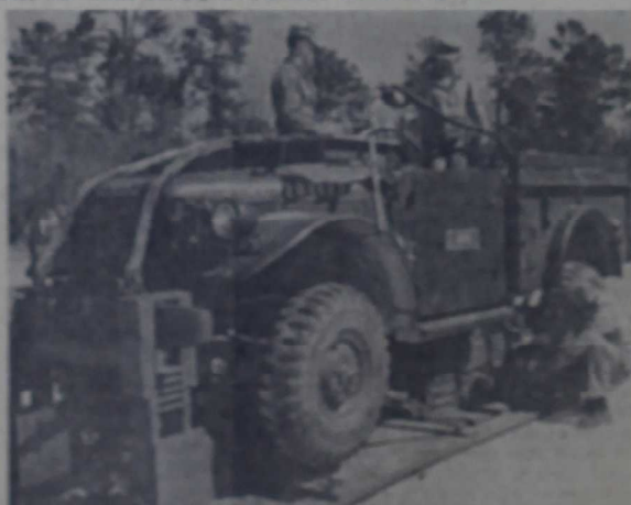
BIG DROP —Capt. N. D. Lapointe, Sgt. A. S. Umphrey, and Capt. J. N. Daley, of Force Troops' 2nd Air Delivery platoon, make final adjustments on the suspension sling and tie-arm straps that will play an important part in safely air dropping a three-quarter ton truck during the air delivery demonstration at Camp Geiger (Official USMC Photo).
