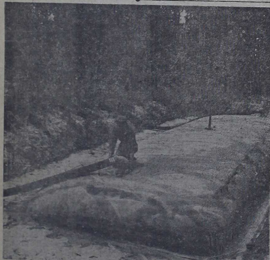
FILL 'ER UP, PLEASE—Pvt. Peter J. Fiocco checks the discharge fitting on a 10,000-gallon tank at the 8th Fuel Co. Tank Farm near Onslow Beach. All fittings must be carefully installed and inspected to avoid damage.
