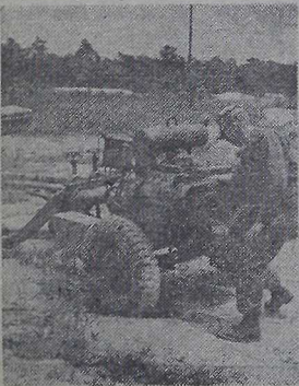
CRANKING OVER—Pfc A. F. Ward starts the pump to begin transfer of fuel to the next station. Each pump is capable of pumping fuel a quarter-mile along, the system to the next pump.
