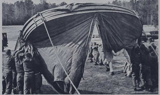
GOING UP—Marines of the 2d Force Service Regiment, Force Troops, demonstrate the "setting-up" of the new Medium Accordion Shelter developed by the Marine Corps Landing Force Development Center, Quantico, Va. (Photo by Sgt. R. F. Messall.)
