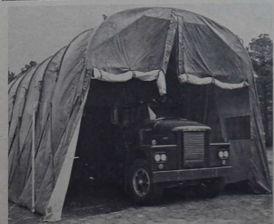
FINISHED—The new Medium Accordion Extendable Shelter, as it looks when it is completely set-up is viewed by Force Troops unit commanders during a display held on March 24 at Harris Field. The shelter was developed by the Marine Corps Landing Force Development Center, Quantico, Va. (Photo by Sgt. R. F. Mescall.) See Page 5 for Story.
