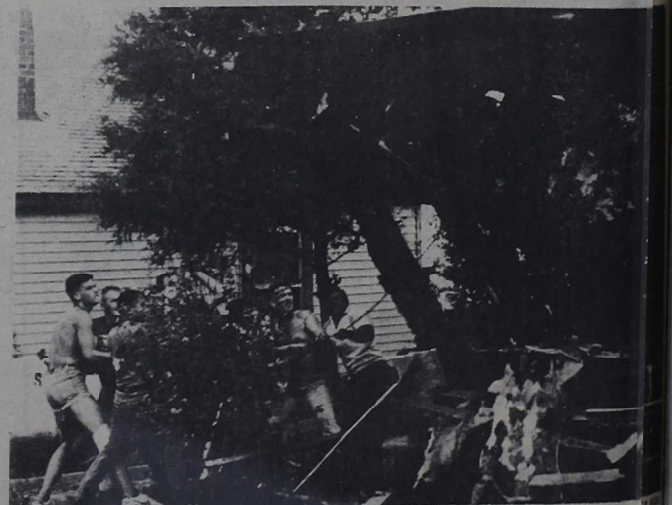
The walls come tumbling down
