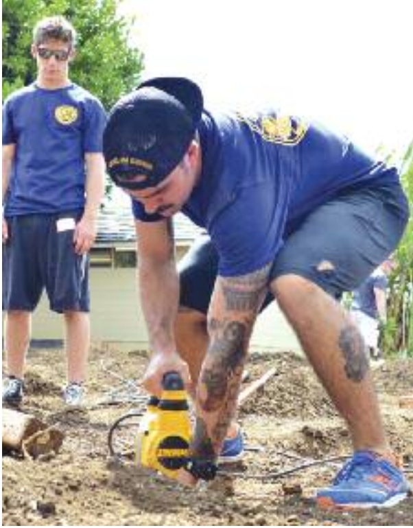
Navy Diver 2nd Class Pierce Decker, Mobile and Diving Salvage Unit One, uses a jackhammer to make room for supporting beams to help hold the new playground for the Holy Nativity School, located in Aina Haina.
