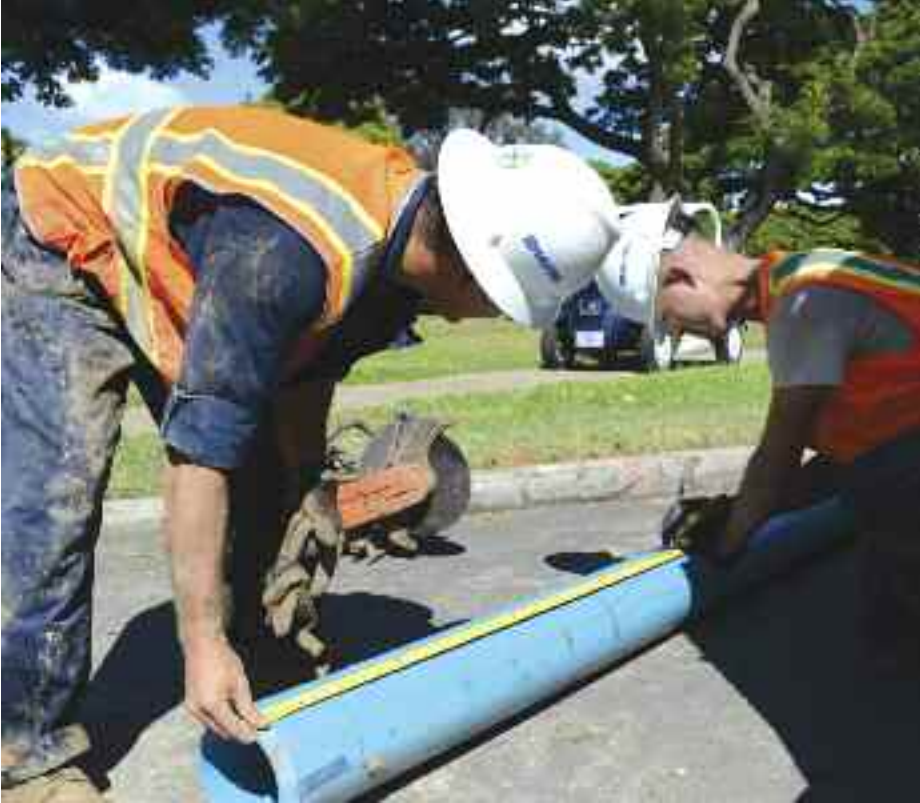
Airman 1st Class Robert T. Shikina, left, a plumber with the 624th Regional Support Group holds the tape measure for Tech. Sgt. Benjamin M. Johnson, right, a plumber with the 647th Civil Engineering Squadron, as he measures off the proper length of PVC pipe needed to replace the cast iron pipe that had sprung a leak.
