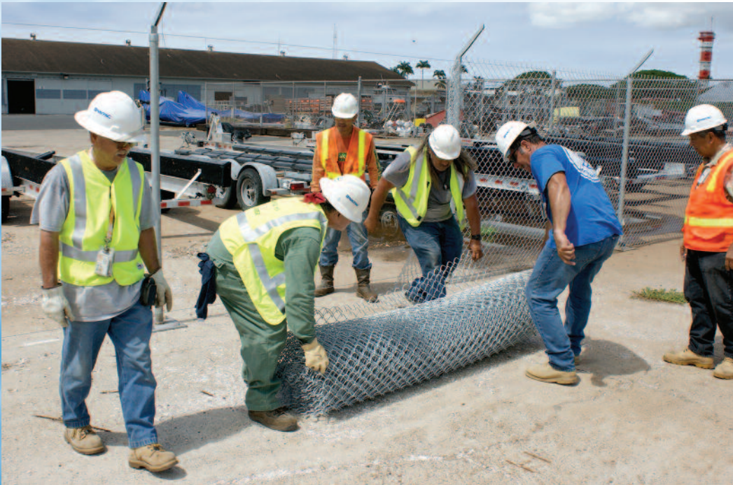
(Above) Naval Facilities Engineering Command (NAVFAC) Hawaii personnel install a security fence with multiple gates around a parking area, including building 5, at Joint Base Pearl Harbor-Hickam at Ford Island, to protect small boat operation's equipment and accessories.
