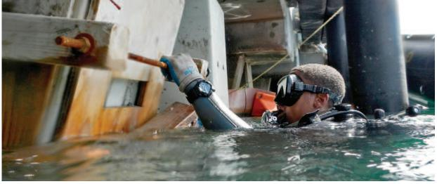
Builder 2nd Class Khiaro Promise from Construction Dive Detachment Alpha, part of Underwater Construction Team 2 (UCT-2) from Port Hueneme, Ca. removes a wood form during a structural pile restoration at the Hotel Piers at Joint Base Pearl Harbor-Hickam. (See additional photos on page A-5.)
