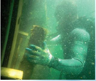
(Above and below) Sailors from Construction Dive Detachment Alpha, part of Underwater Construction Team 2 (UCT-2) from Port Hueneme, Calif. remove wood forms during a structural pile restoration at the Hotel piers at Joint Base Pearl Harbor-Hickam. (See story on page A-6)
