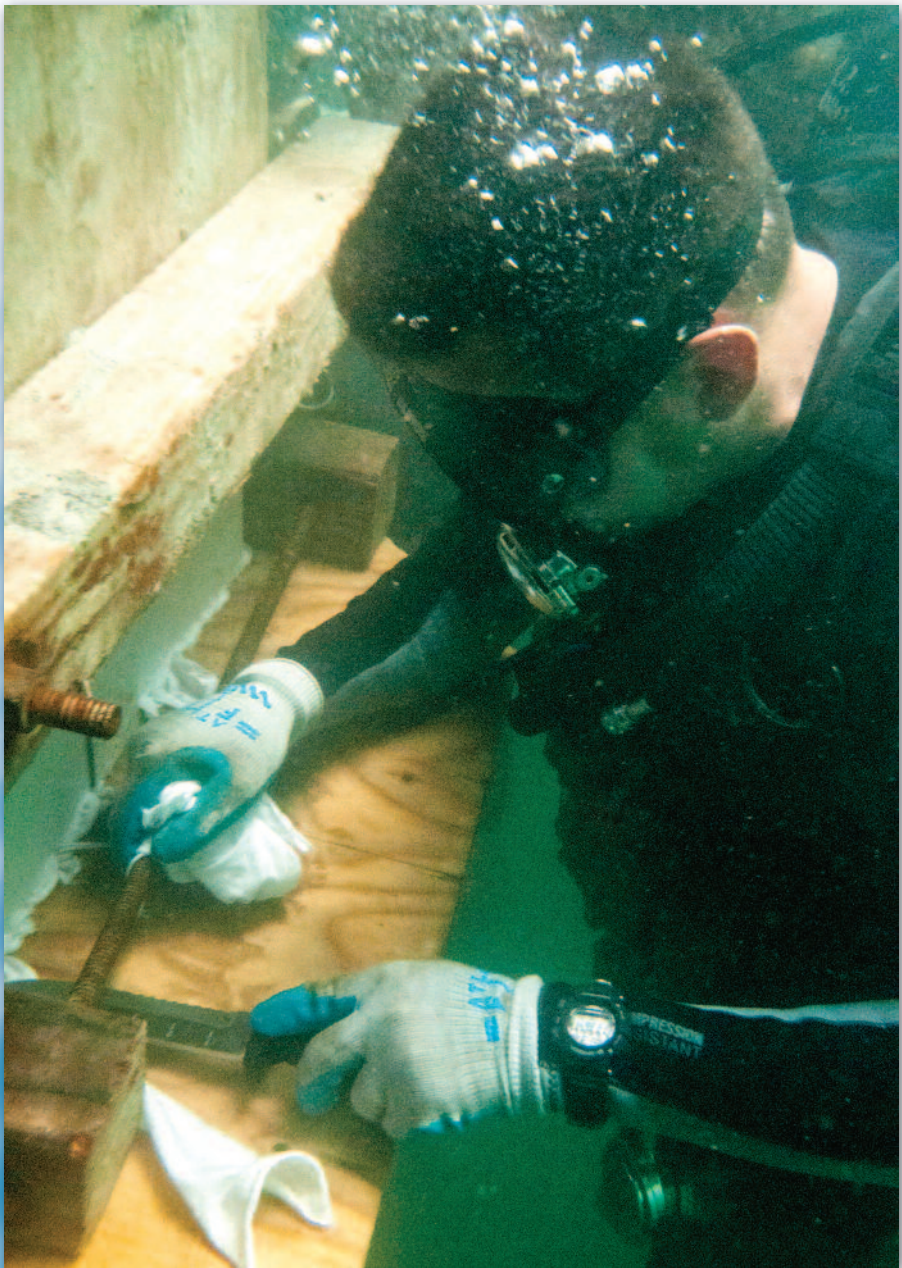
Builder 2nd Class Keith Reed from Construction Dive Detachment Alpha, part of Underwater Construction Team Two (UCT-2) from Port Hueneme, Calif. works during a structural pile restoration at the Hotel piers on Joint Base Pearl Harbor-Hickam. The underwater construction team provides a capability for construction, inspection, repair, and maintenance of ocean facilities in support of Navy and Marine Corps operations.
