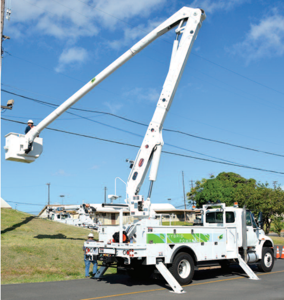
Naval Facilities Engineering Command (NAVFAC) Hawaii utilities personnel use the new hybrid bucket truck in the field for the first time. Power lines between multiple poles on the command's main compound were replaced at Joint Base Pearl Harbor-Hickam.
