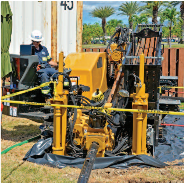
An employee from contractor AECOM operates a horizontal drill rig June 10 that will install a soil vapor extraction (SVE) system at Onizuka Village housing at Joint Base Pearl Harbor-Hickam.
