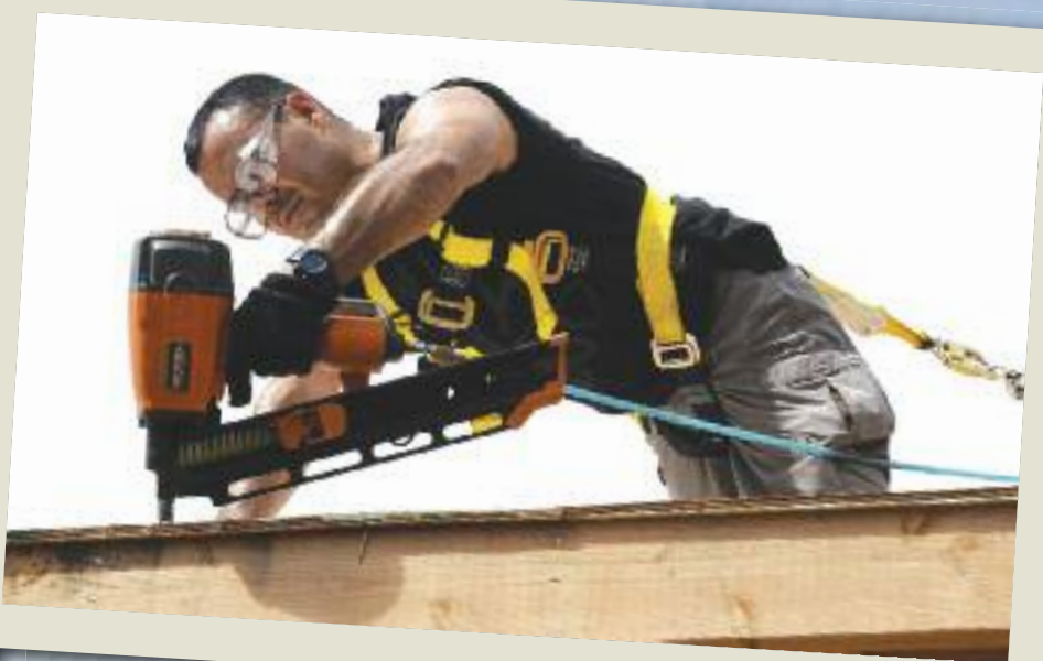
Tech. Sgt. Manny Garibay, 15th Maintenance Group, uses a nail gun to secure plywood on a rooftop.
