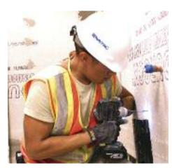
As part of the Hickam Gymnasium's foyer bathrooms complete makeover, an Air Force apprentice installs cement backer board to the walls of the men's restroom at Joint Base Pearl Harbor-Hickam.
