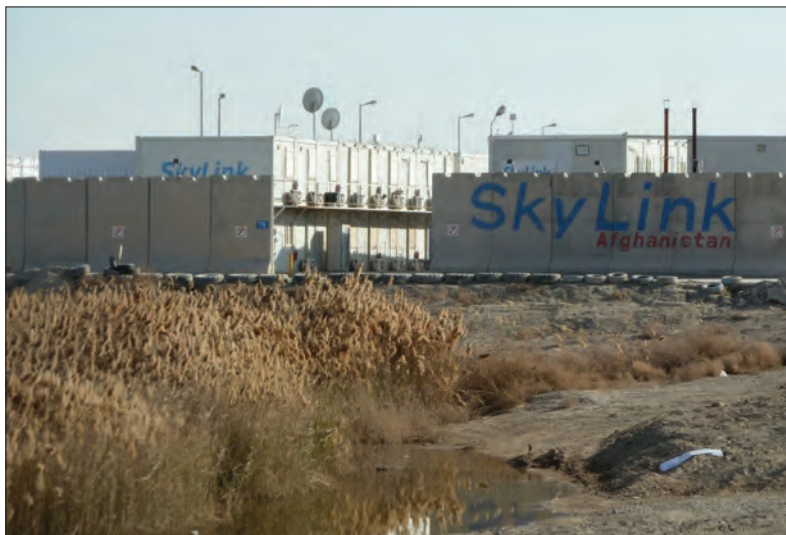
▲ Thousands of these site assembled structures of relocatable buildings in Afghanistan are put together with insulated steel interlocking panels placed on a concrete slab. The buildings, with showers and toilets, are a luxury compared to tents with an accessory latrine and shower building.
