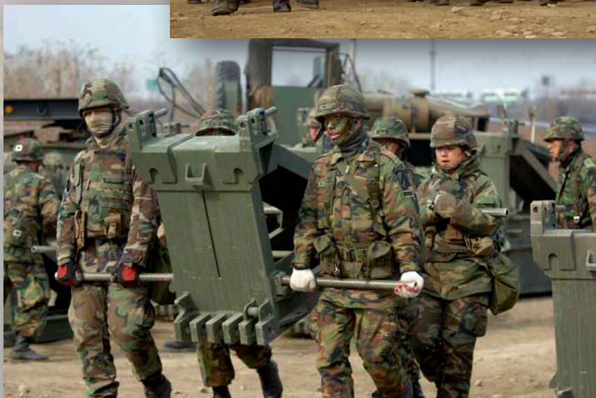
Above: Seabees from NMCB 5 work with members of the ROK 11/75th Bridge Seoul Construction Co. as they move a 700-pound transom beam.
