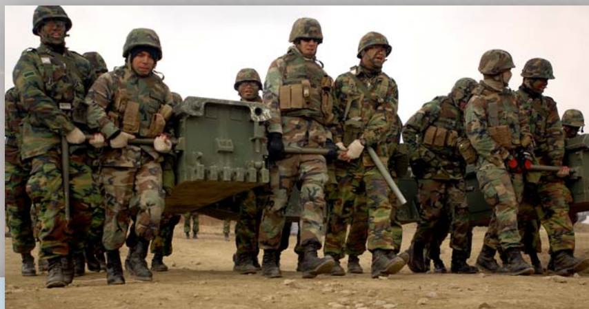
Above: Seabees from NMCB 5 work with members of the ROK 11/75th Bridge Seoul Construction Co. as they move a 700-pound transom beam.
