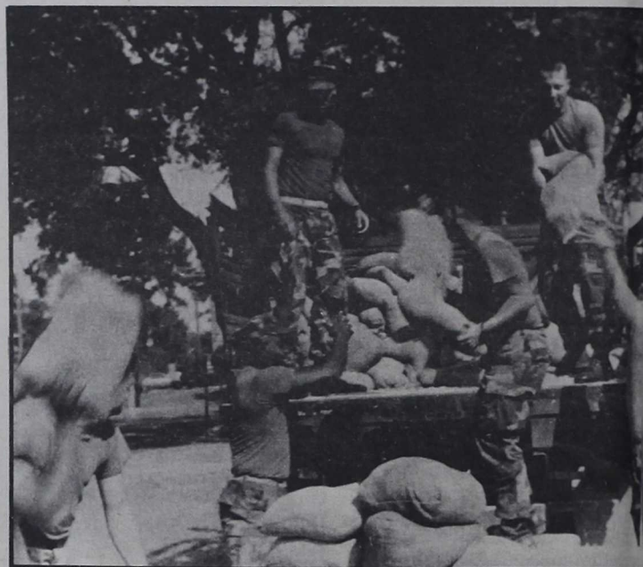
Marines load sandbags onto a truck after the operation at Building 1 was completed to build the bunkers around the building.
