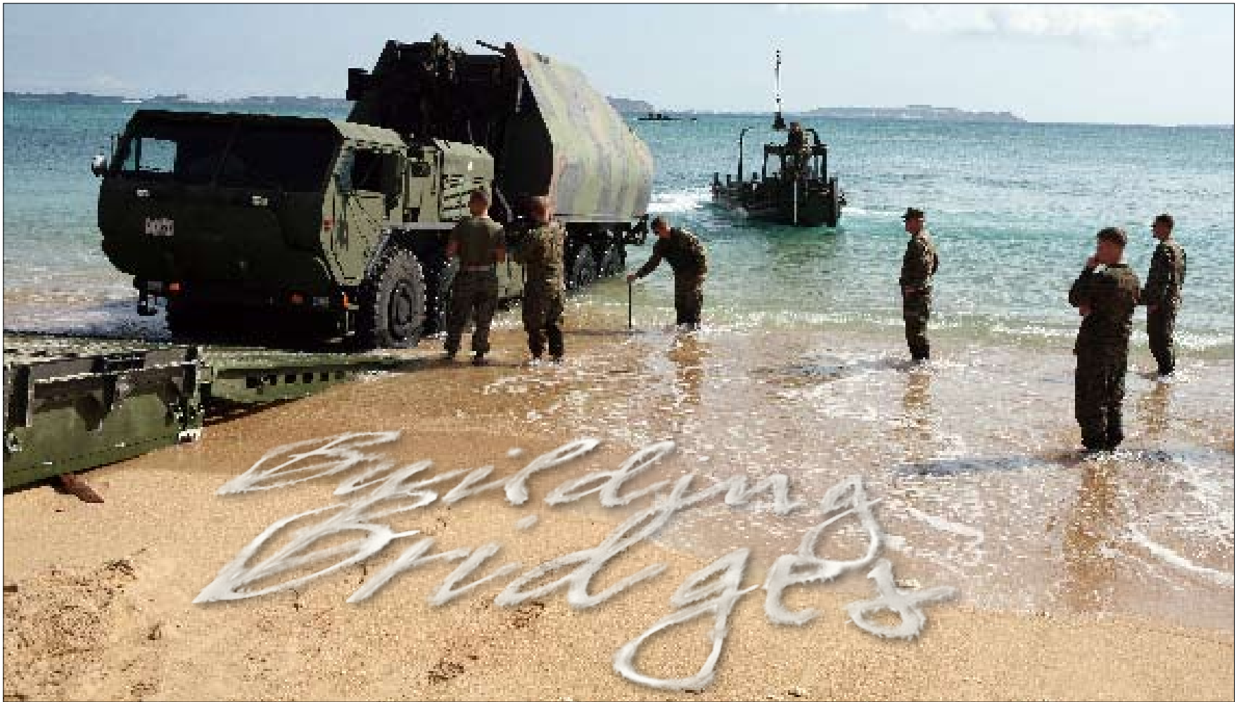
Marines with Company A, 9th Engineer Support Battalion, 3rd Marine Logistics Group, III Marine Expeditionary Force, launch an improved ribbon bridge from a medium girder bridge into the waters off Kin Blue beach during military occupational specialty training recently. Photo by Lance Cpl. Antwain J. Graham
