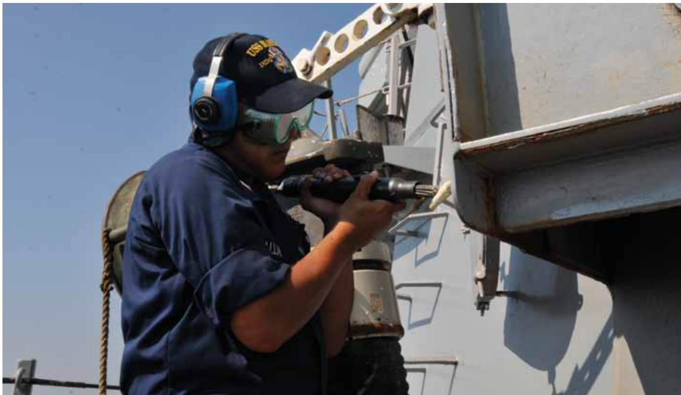
▲ Boatswains Mate 2nd Class (AW/5W) William Magallanes, from New Port News, Va., uses a needle gun to remove the rust and old paint from the hull of the USS Mahon (DDG 72). U.S. Navy photo by Mass Communication Chief William Lovelady.
